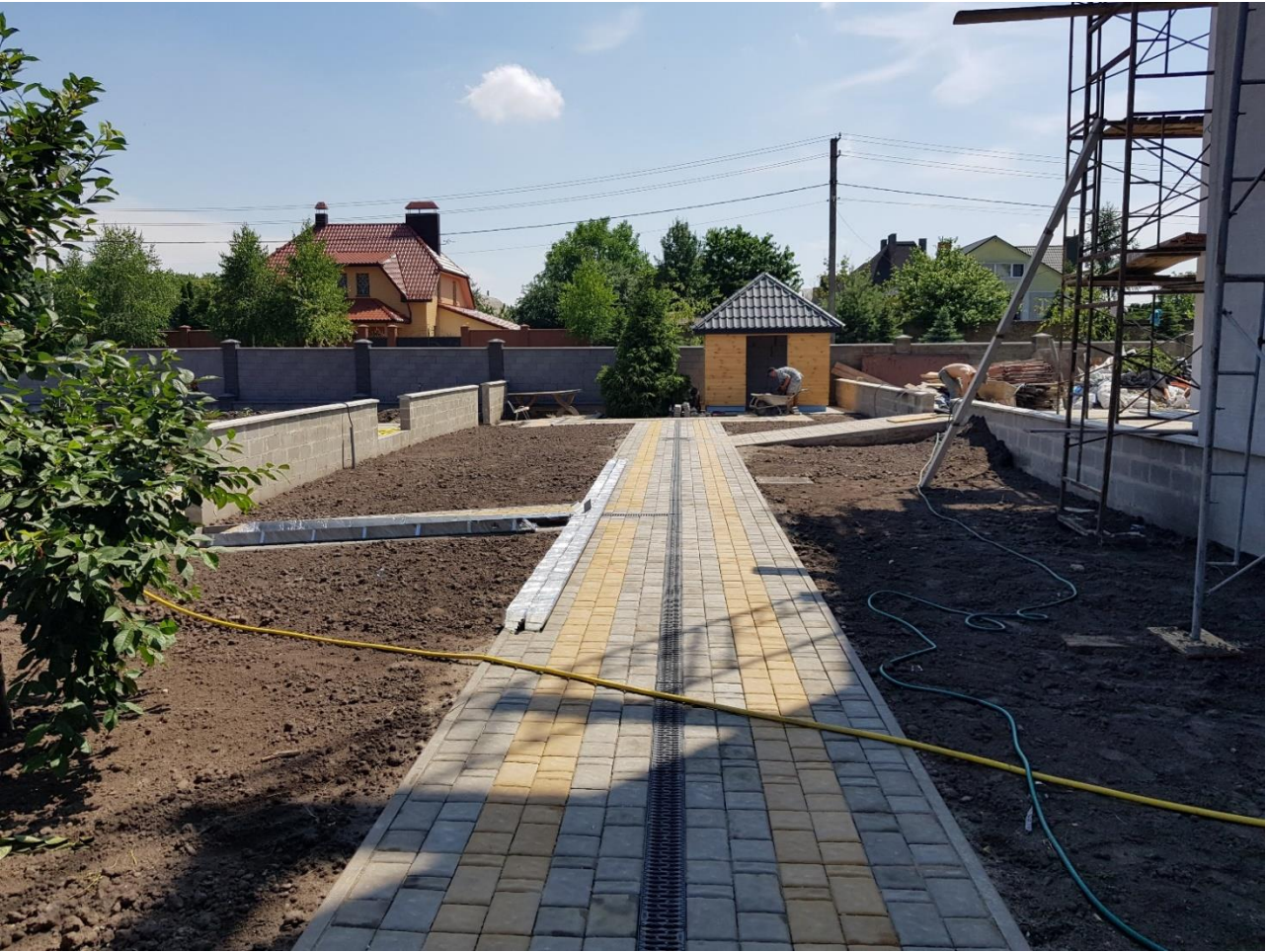
Paving stones being laid.
